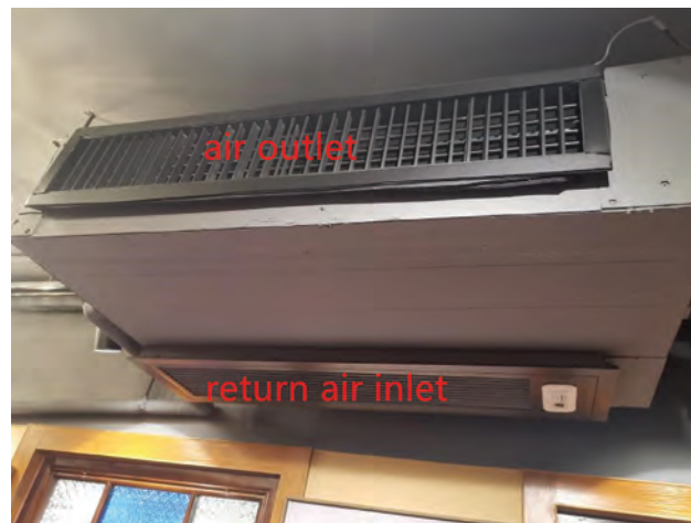
Figure 1. Inlet and outlet of air conditioner described in study of COVID-19 outbreak associated with air conditioning in restaurant, Guangzhou, China, 2020 (2).
