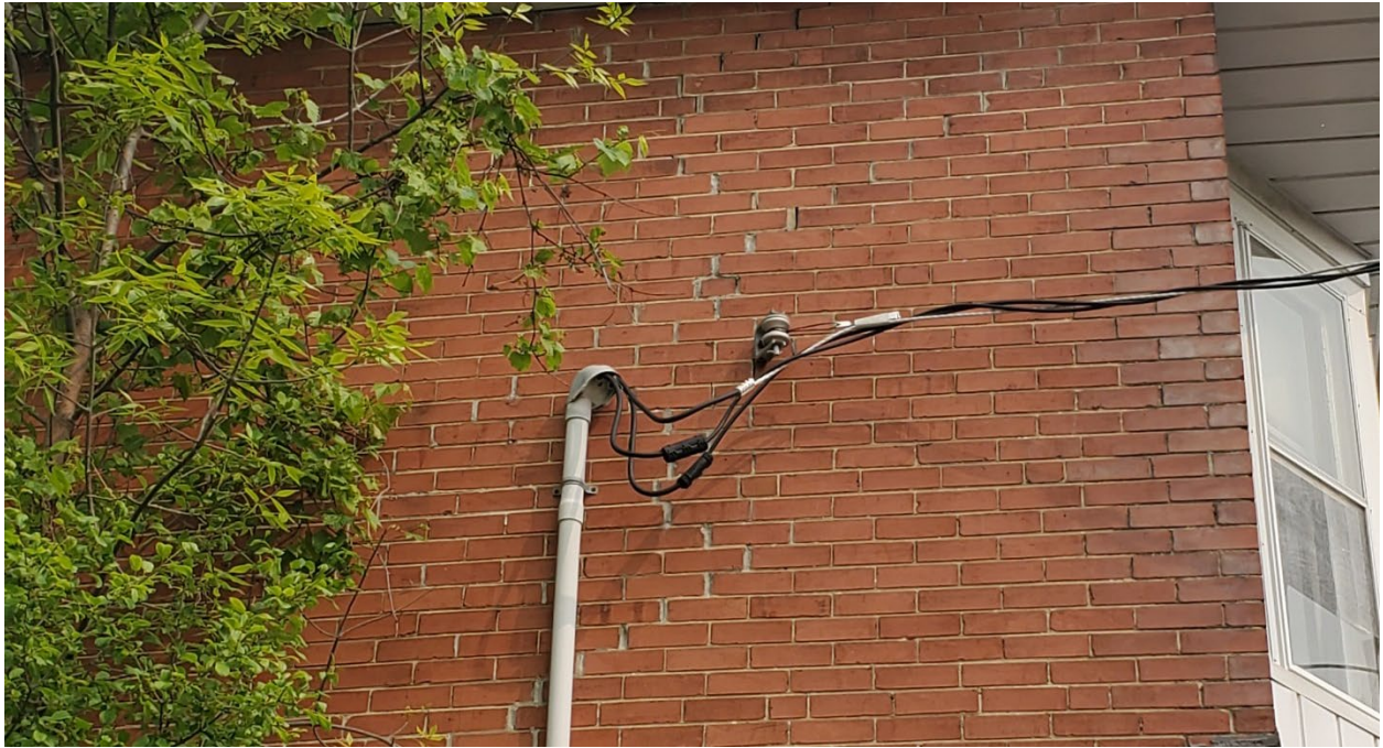
Photo 16. View northwest of the atypical common bond brick pattern on the south elevation of the building
