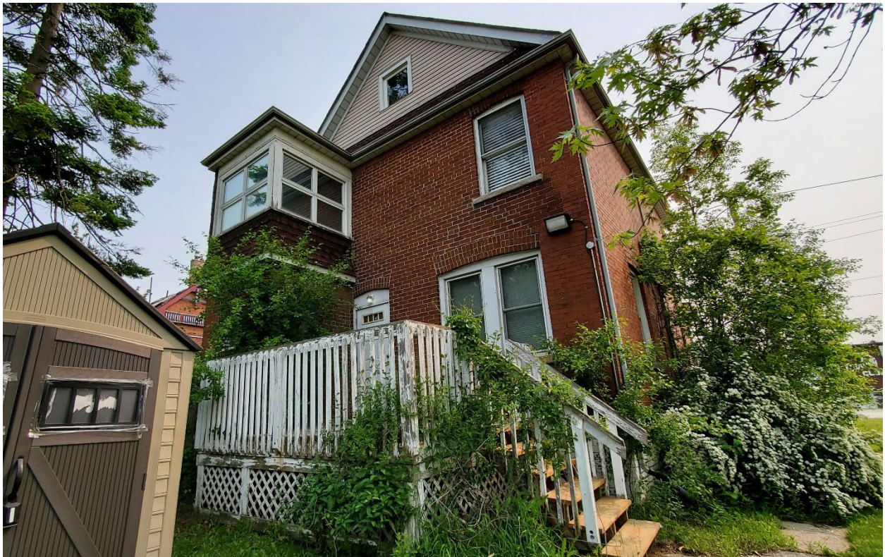
Photo 17. View northeast of the common bond brick pattern comprising most of the west elevation of the building
